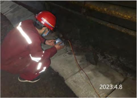
A worker wearing a red jacket with reflective stripes and a red helmet is kneeling on the ground at night, testing a ground connection. The worker is holding a testing device with red and black cables. A timestamp '2023.4.8' is visible in the bottom right corner of the photo. |
