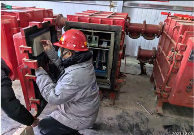
A photograph showing a worker in a grey jacket and red helmet inspecting a high-voltage vacuum circuit breaker. The worker is kneeling and looking at the internal components of the device. The device is red and has a black door open. The background shows other similar devices in a room. A timestamp '2023.12.09' is visible in the bottom right corner of the photo. |
